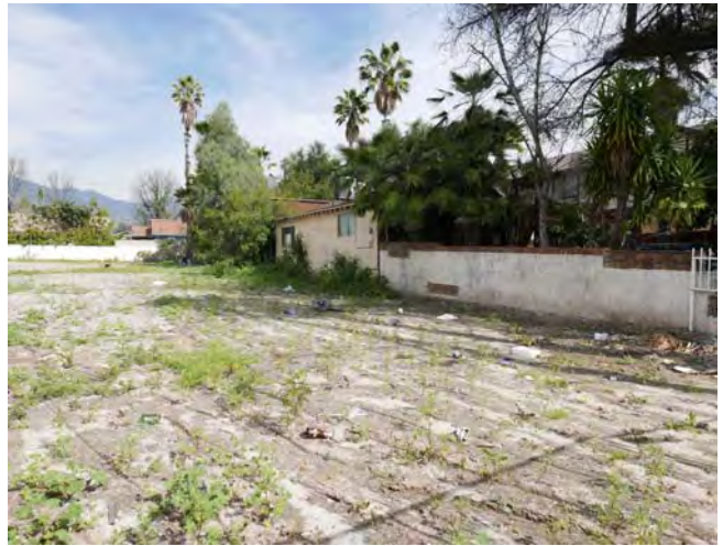
View of the western façade
