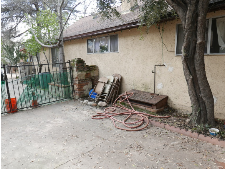
Figure 5: Secondary (Eastern) Façade, 715 W. Duarte Road SOURCE: Sapphos Environmental, Inc., 2017
