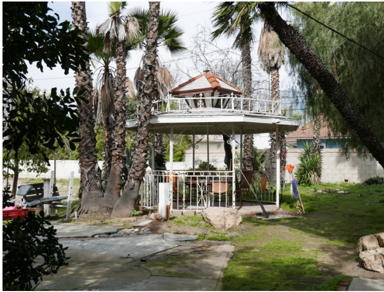
Figure 9. Gazebo, 715 W. Duarte Road SOURCE: Sapphos Environmental, Inc., 2017
