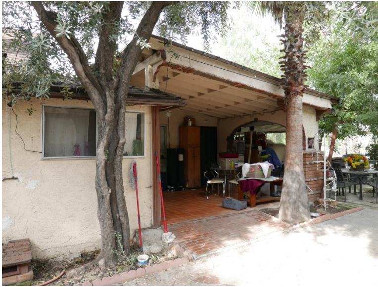
Figure 7. Patio, 715 W. Duarte Road SOURCE: Sapphos Environmental, Inc., 2017
