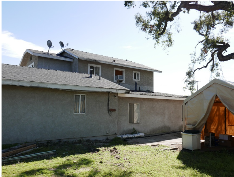
Figure 7. Tertiary (Western) Façade, 146 E. Cherry Avenue SOURCE: Sapphos Environmental, Inc., 2017
