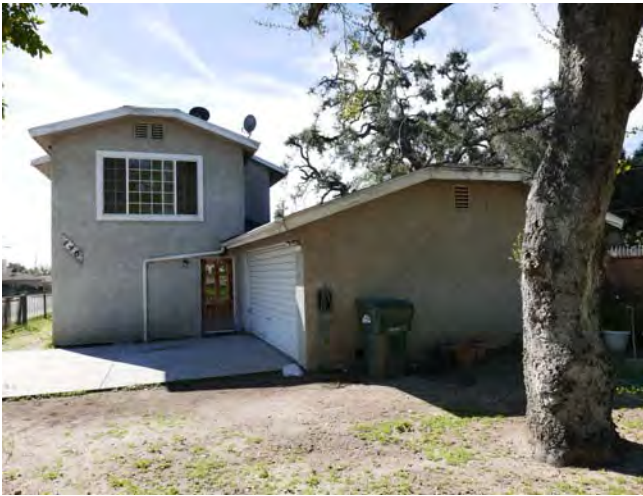
View of the northern façade
