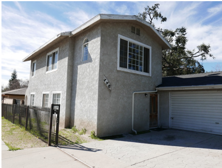
Figure 4. Primary Façade, 146 E. Cherry Avenue SOURCE: Sapphos Environmental, Inc., 2017
