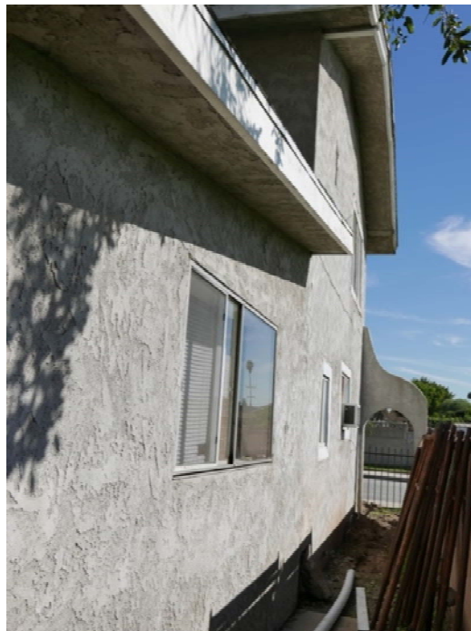
Figure 6. Secondary (Southern) Façade, 146 E. Cherry Avenue SOURCE: Sapphos Environmental, Inc., 2017
