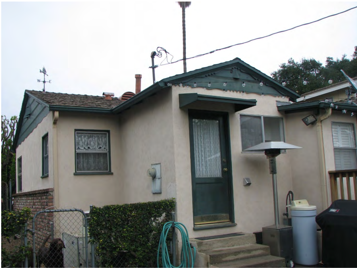
Calvin Smith House, rear porch, 616 E. Foothill Boulevard, February 3, 2016 (Charles J. Fisher photo)
