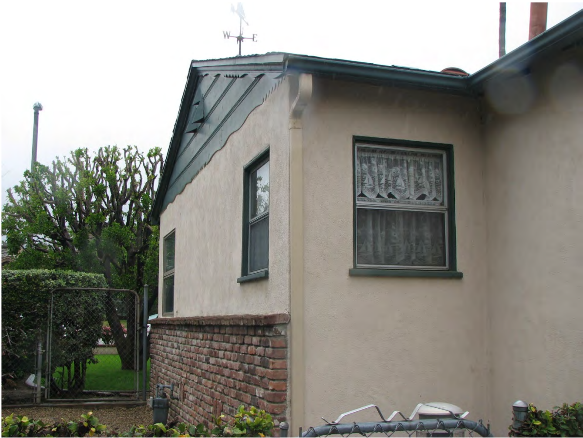
Calvin Smith House, West wing and gable, 616 E. Foothill Boulevard, February 3, 2016 (Charles J. Fisher photo)
