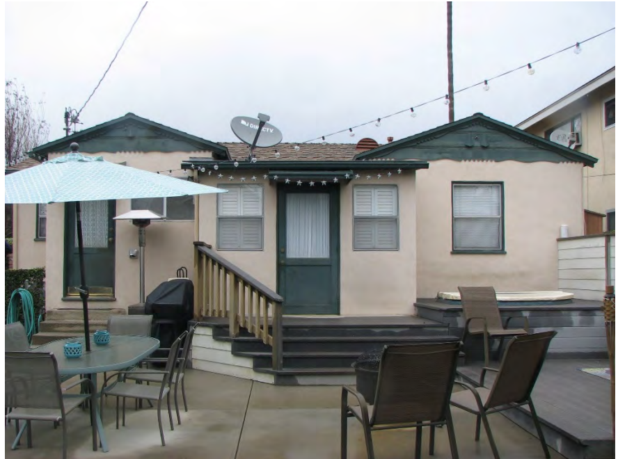
Rear façade of the Calvin Smith House showing the 1993 family room extension between the two small rear wings of the house.
