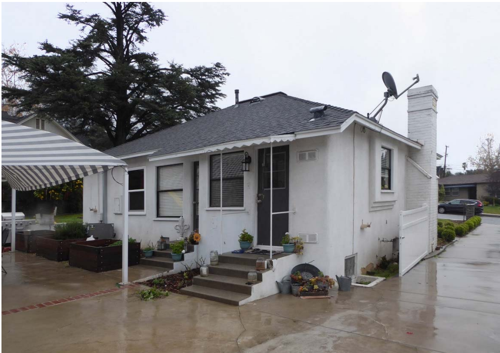
Figure 9. View of the southwest oblique looking northeast.
