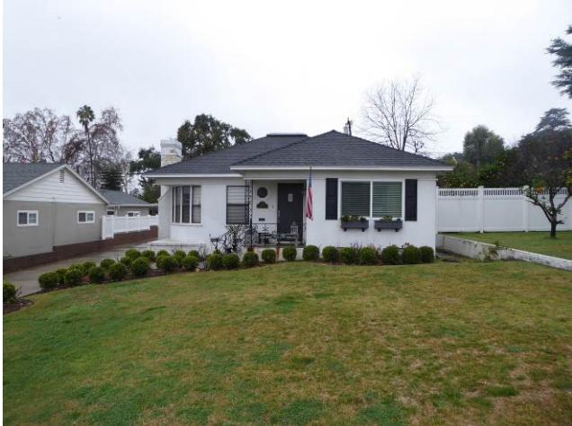
Image 1. View of the primary (east) facade looking west.
