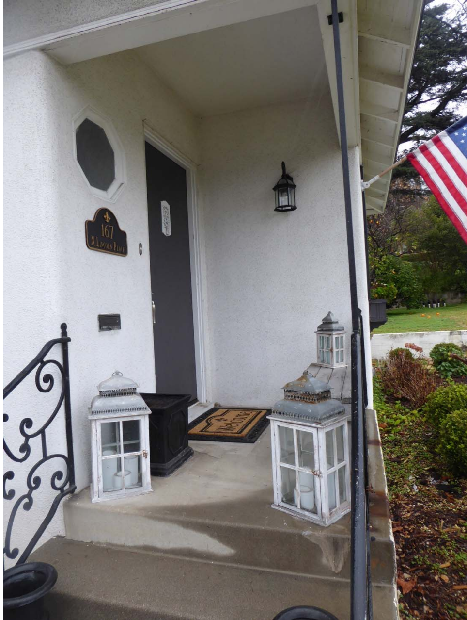
Figure 6. Detail of the porch and primary entrance.
