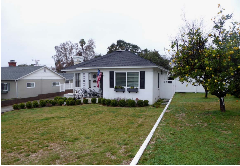
Figure 5. View looking southwest at the northeast oblique of the house.
