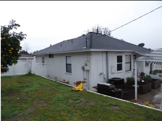
Image 3. View of the northwest oblique looking southeast.
