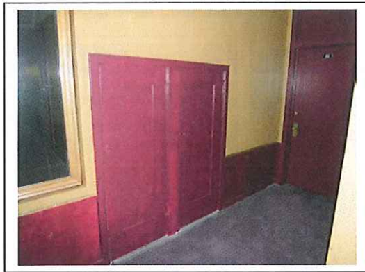
Figure 144 – Apartment Kitchen access doors, 2006
