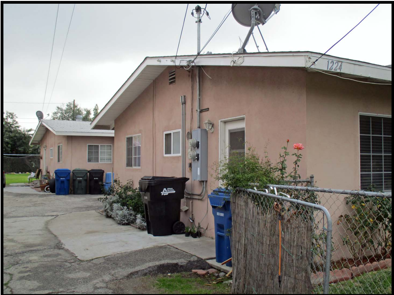
North Elevation of West Unit, 1224 S. Alta Vista Avenue, Monrovia, CA (SE)
