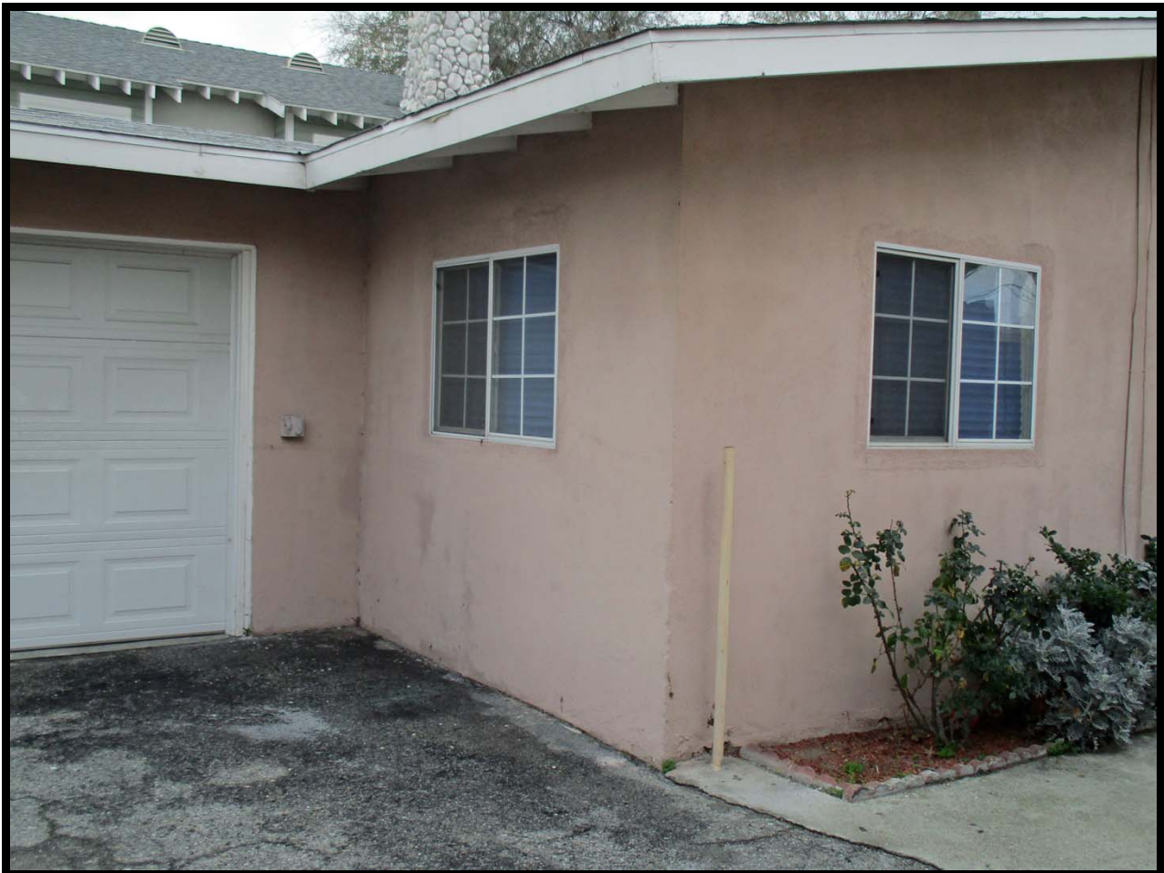
South Elevation, West Unit, 1224 S. Alta Vista Avenue, Monrovia, CA (SW)
