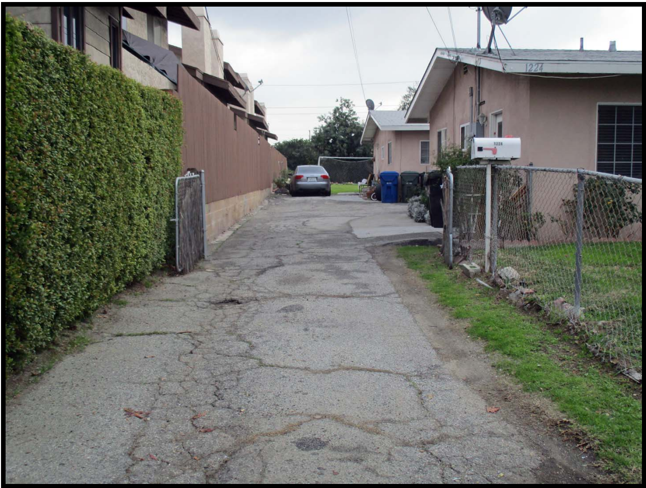
Driveway at 1224 S. Alta Vista Avenue, Monrovia, CA (E)
