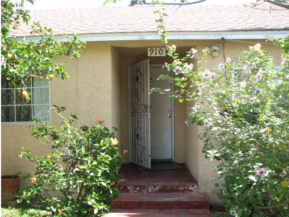
The Miller Houses, front porch of front house, 910 S. Ivy Avenue, April 6, 2017 (Charles J. Fisher photo)
