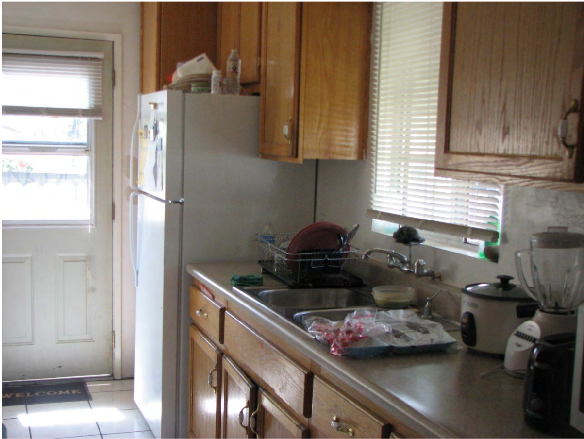
The Miller Houses, kitchen in rear house, 910½ S. Ivy Avenue, April 6, 2017 (Charles J. Fisher photo)
