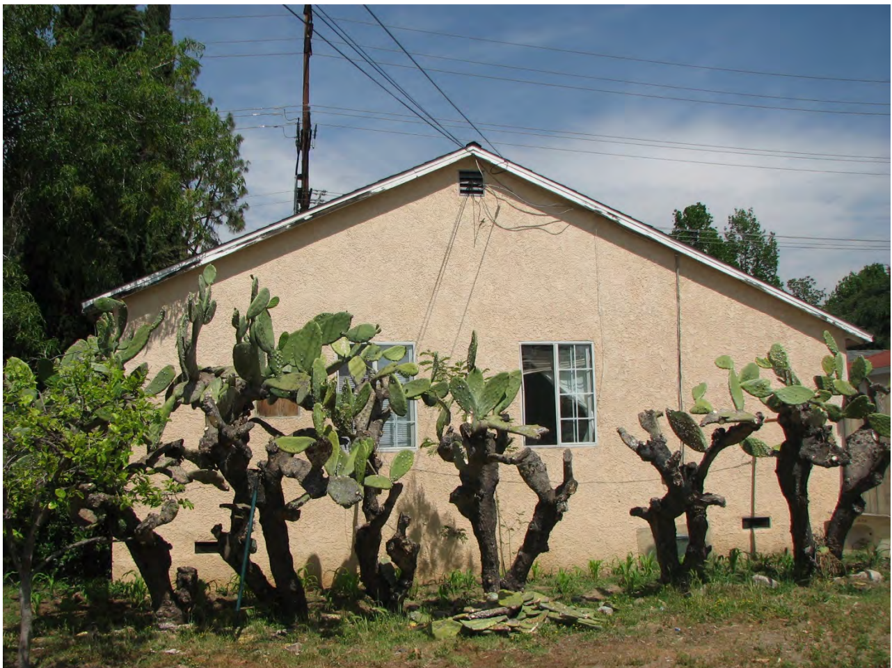
The Miller Houses, South façade of front house, 910 S. Ivy Avenue, April 6, 2017 (Charles J. Fisher photo)
