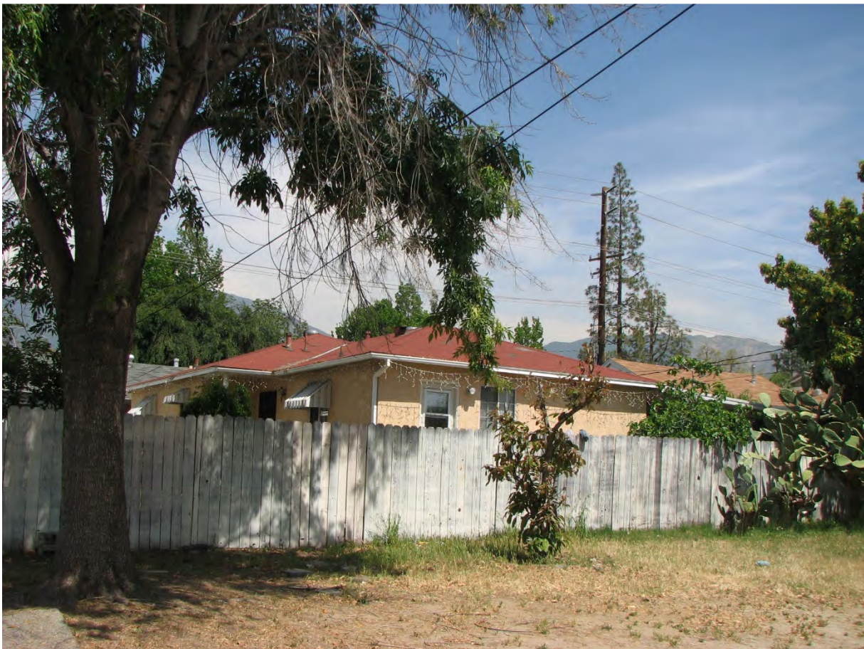
The Miller Houses, rear house behind fence, 910½ S. Ivy Avenue, April 6, 2017 (Charles J. Fisher photo)
