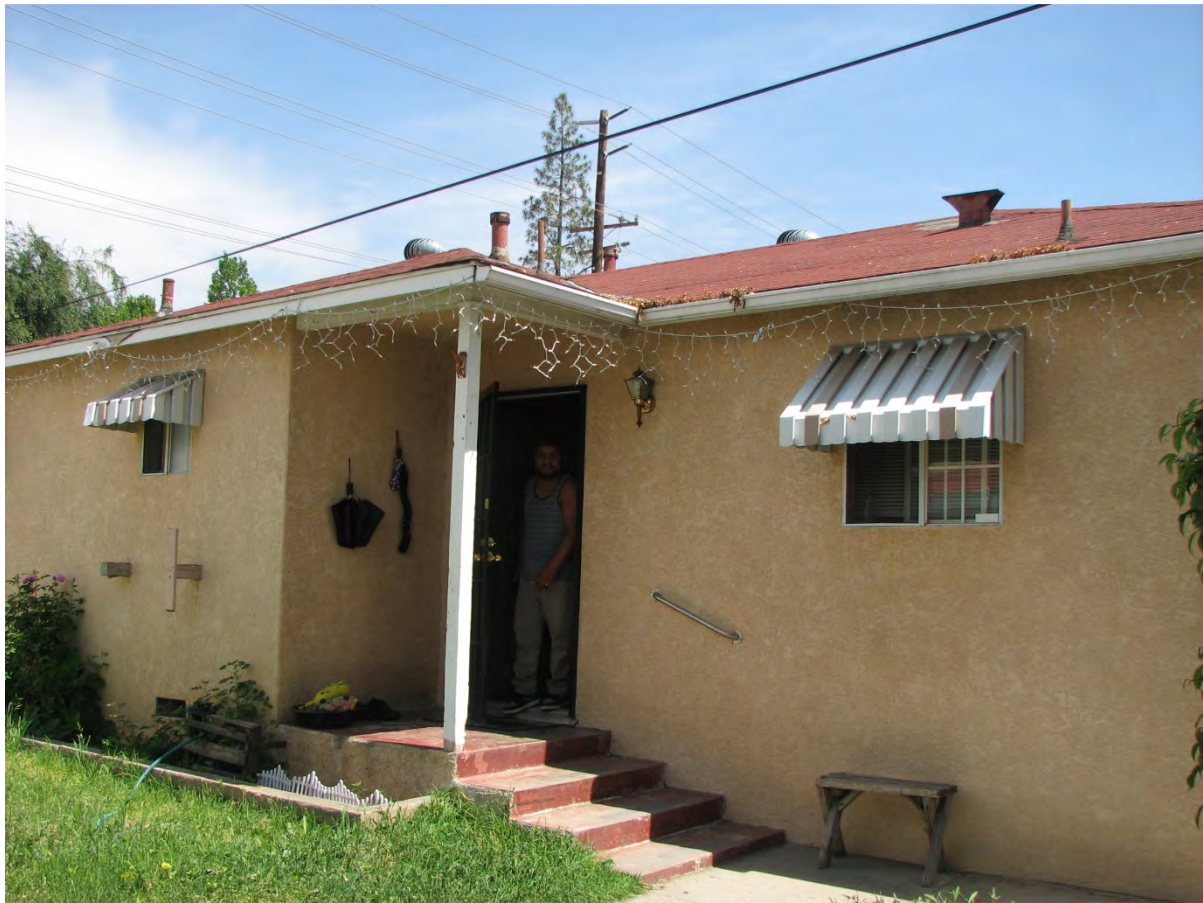
The Miller Houses, rear house, 910½ S. Ivy Avenue, April 6, 2017 (Charles J. Fisher photo)
