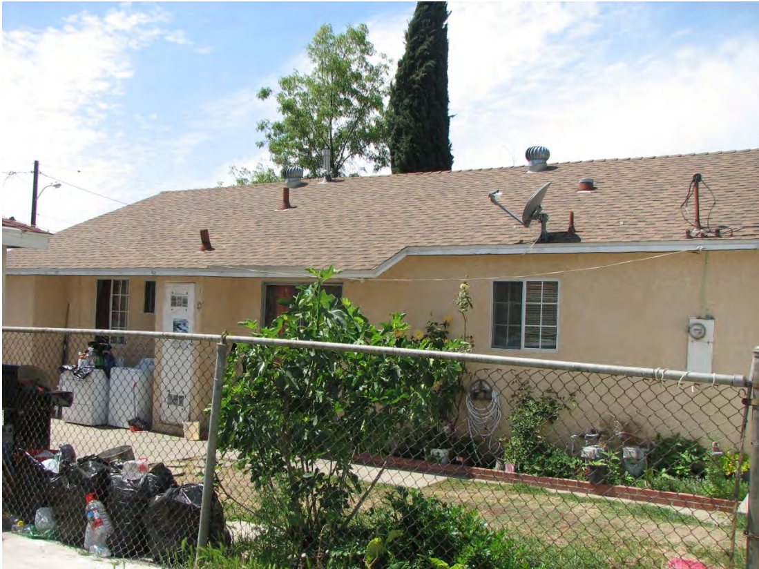
The Miller Houses, rear façade of front house, 910 S. Ivy Avenue, April 6, 2017 (Charles J. Fisher photo)
